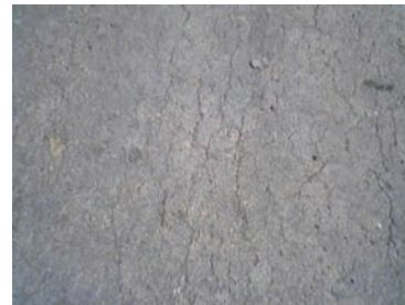
Control - Stripped asphalt surface with cracks and depression
