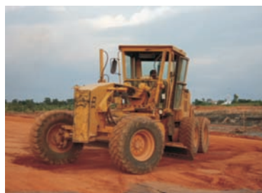
Soil surface levelling
