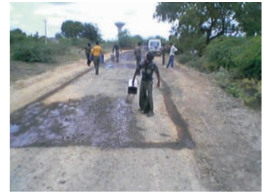
Prime coat - Terrasil with cationic bitumen emulsion
