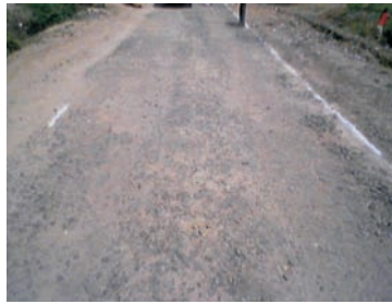
Compacted WBM after two compacted soil layer
