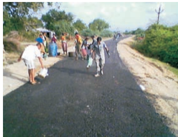
Tack coat – Nanotac with cationic bitumen emulsion
