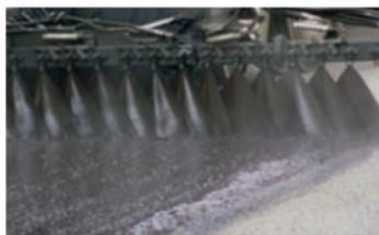
With Nanotac - Clean nozzles. Uniform spraying at 40 – 50 °C
